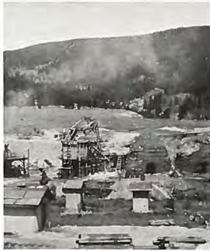
View of the gravel crushing outfit used in furnishing material for surfacing one of the early Tennessee Pass projects.
