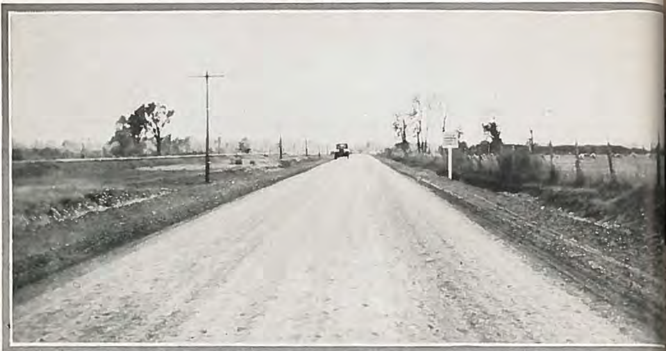
"Mixed in place" oil surfaced Federal Aid highway south of Alamosa.
