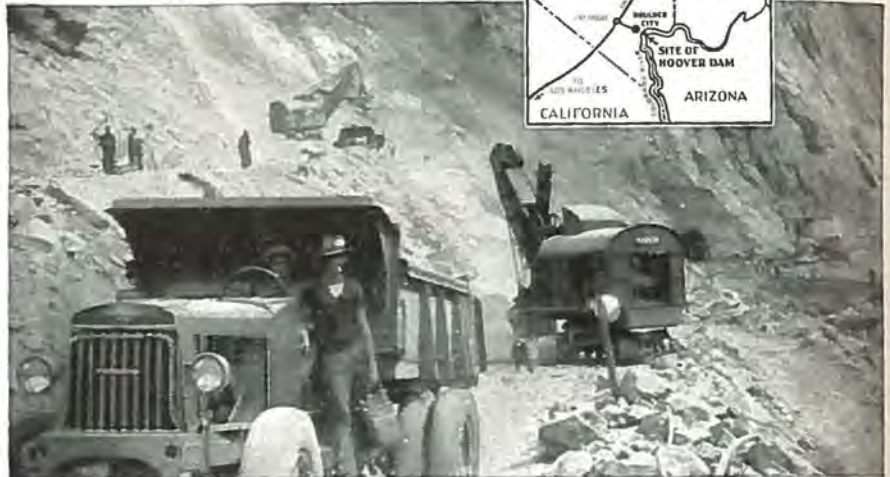
One of the International heavy-duty trucks working at Hoover Dam. The open hood is expressive of the intense heat in the canyon, rising as high as 128 degrees. The boulder-proof armored cab is further evidence of conditions encountered. Note, at right of shovel, the entrance to an auxiliary tunnel used in construction of the great diversion tunnels that will extend three miles through solid rock.
