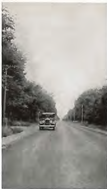
Another example of Federal Aid road construction in Colorado—an oil-surfaced highway in Fremont County.
