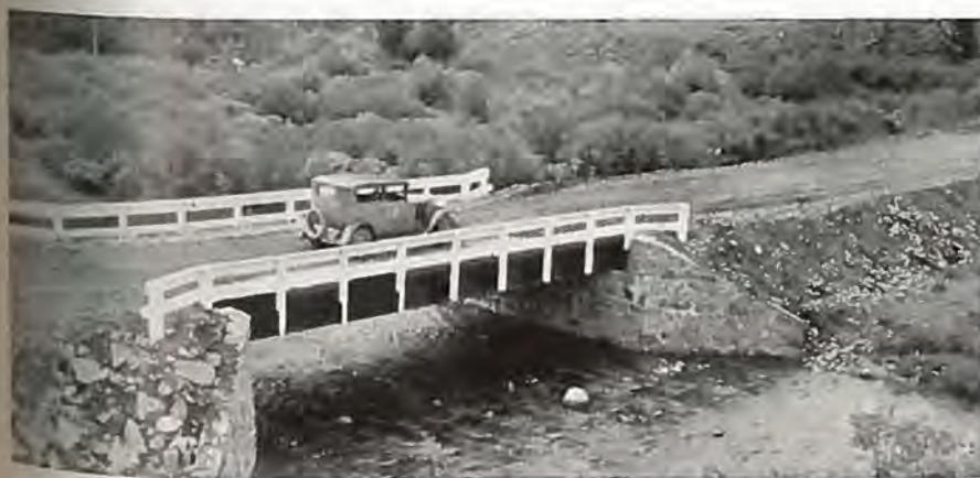
One of the standard log crib timber bridges constructed as a part of the project. Headwalls are of cement rubble masonry.
