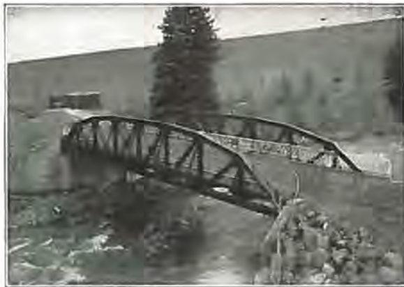
100 ft. Riveted Low Truss Span, Dillon, Colo.
