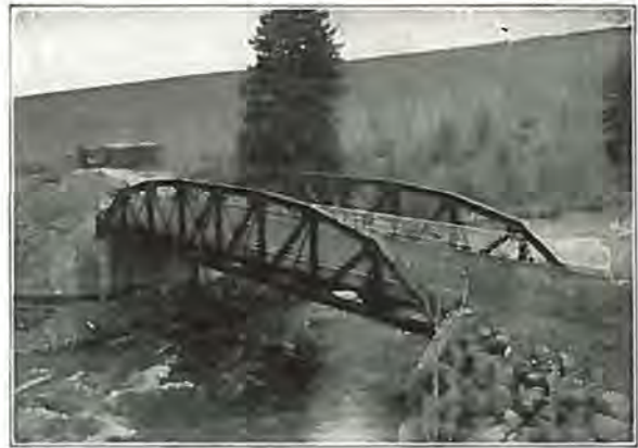
100 ft. Riveted Low Truss Span, Dillon, Colo.
