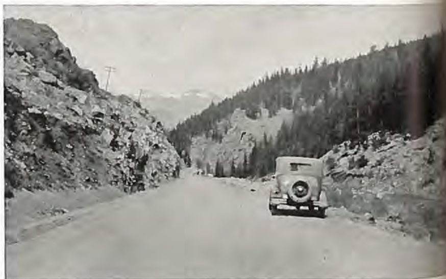
A section of the newly completed standard Federal Aid highway on Kenosha pass in Park county, constructed by the State Highway Department, eliminating the steep grade between Denver and the western slope. The old grade over this two-mile section was almost prohibitive in low for most cars.
