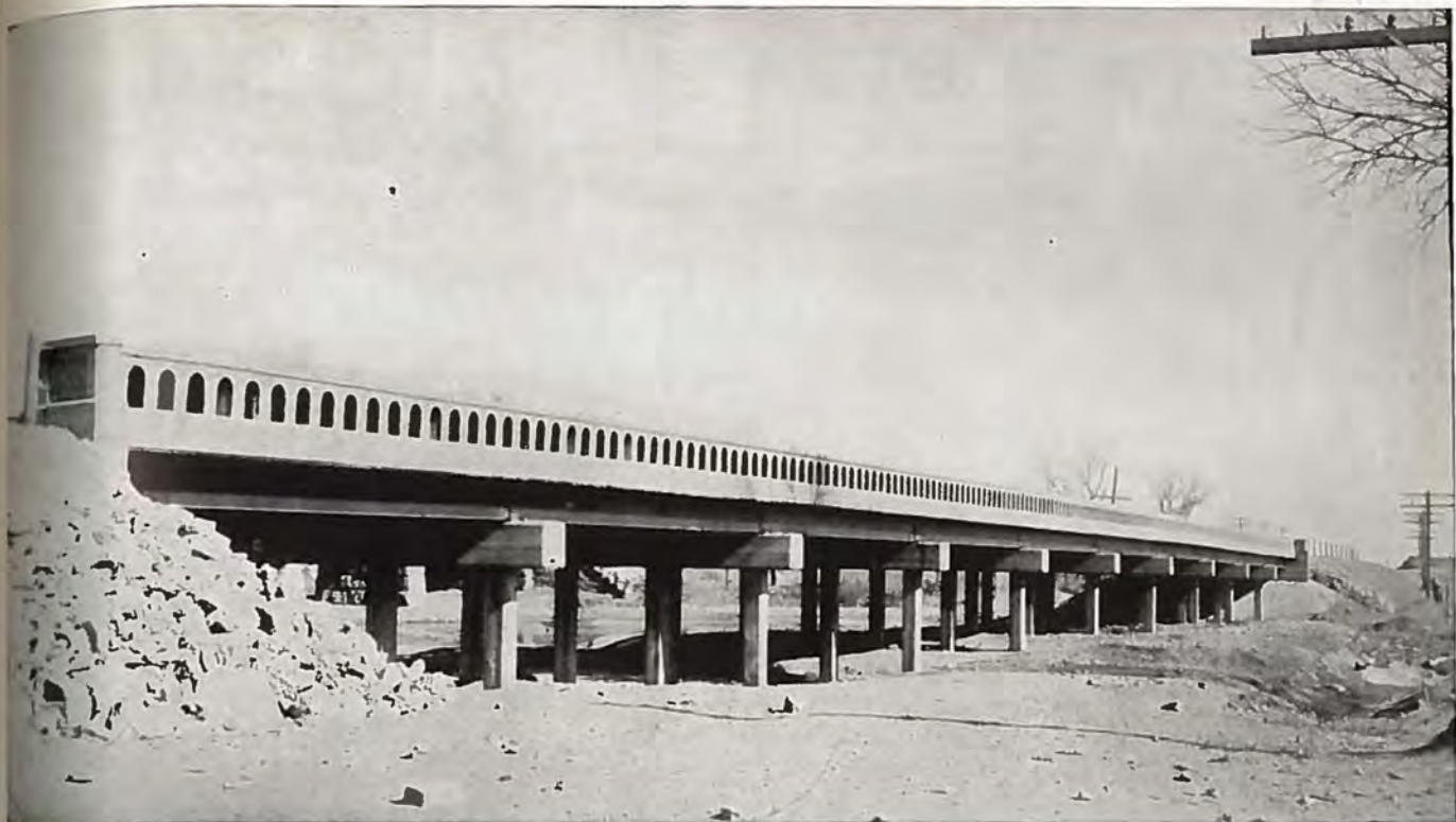
The new Colorado highway bridge over Clay Creek, located east of Lamar, is of reinforced concrete pile trestle type construction. Ideal Cement was used exclusively. It was designed under the supervision of Paul M. Bailey, Bridge Engineer, State Highway Department. The Division Engineer was James D. Bell of Pueblo and the contractor, W. A. Colt & Son, Las Animas, Colorado. The Resident Engineer was L. A. Rose of Pueblo.
