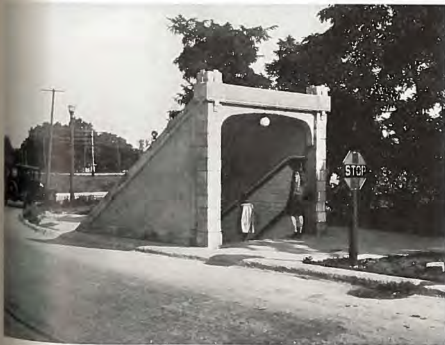
Pedestrian subway, crossing Center Street, Chicago. Two sets of railroad tracks are crossed by the subway.
