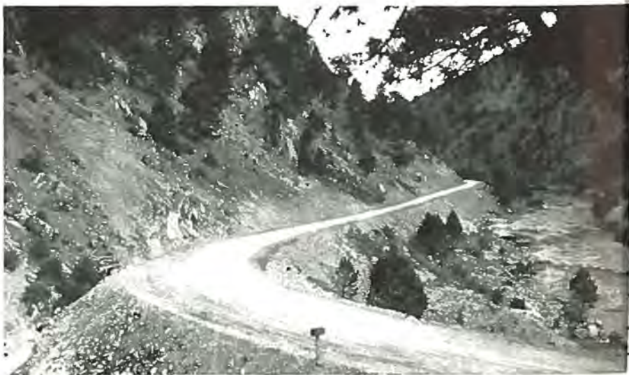
A link of the Decker Springs-Buffalo highway recently completed by the U. S. Bureau of Public Roads in the Pike National Forest. This road is heavily traveled by tourists and sportsmen during the summer months.
