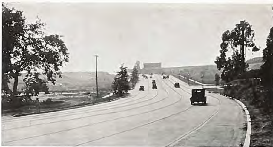
Wellshire Boulevard in Los Angeles, one of the heaviest traveled streets in the world, showing six lanes for traffic with eight-foot parking strips on each side.
