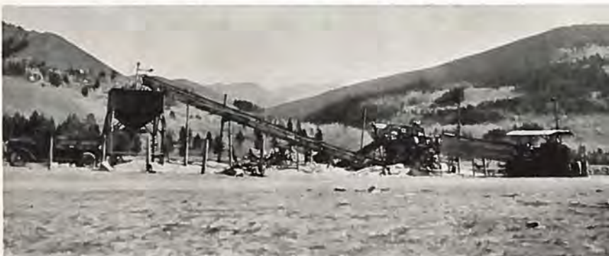
A Pioneer gravel crushing outfit preparing surfacing material for ten miles of new grading on Tennessee Pass, near Redcliff.
