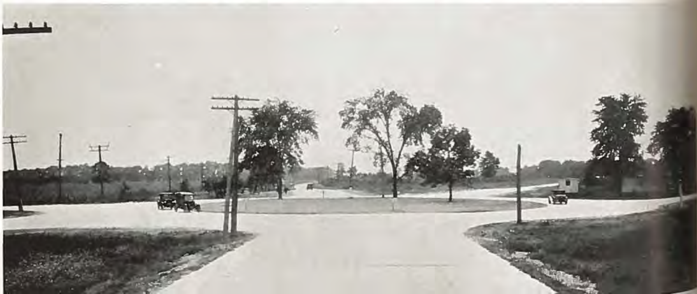
One of the newly designed traffic circles recently completed in Wayne County, Michigan.
