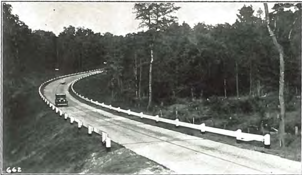
Embankment and curve protected by Resiliflex Road Guard
