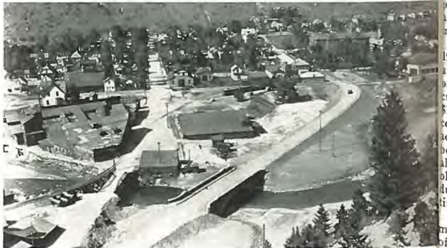
View of bridge and new road in Idaho Springs, connecting with the famous Chicago Creek-Mt. Evans highway, constructed by U. S. Bureau of Public Roads.
