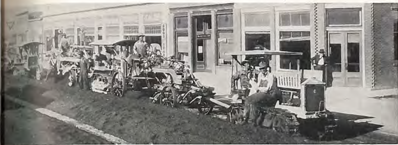
A battery of tractors and graders mixing oil surfacing material on state route through the city of Antonito. Photo by Jackson Studio through courtesy Antonito Chamber of Commerce.
