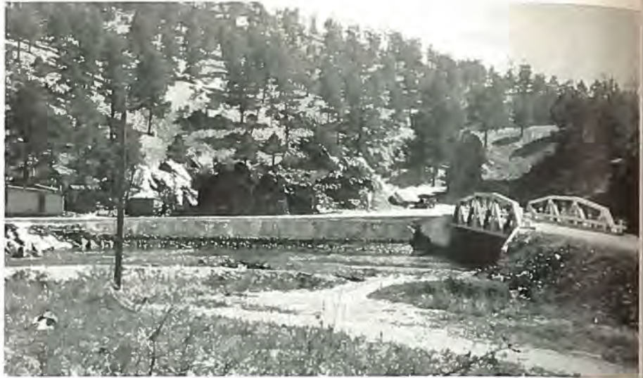
Showing newly constructed Forest highway at Decker Springs, with bridge over South Platte River, forming a part of the network of roads in the Pike National Forest. Photo by U. S. Bureau of Public Roads.
