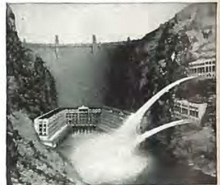
Hoover Dam as it will look on completion, towering 730 feet above foundation rock, with power houses on both banks of the river. The dam will be nearly 1200 feet long, 45 feet thick at the top, and 650 feet thick at the base. This barrier will form a reservoir 115 miles in length with a shore line of 550 miles and an area of 227 square miles, the largest artificial lake in the world.
