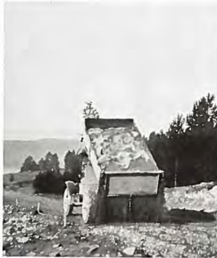
Dumping base course of crushed gravel on roadway near Station 442.
