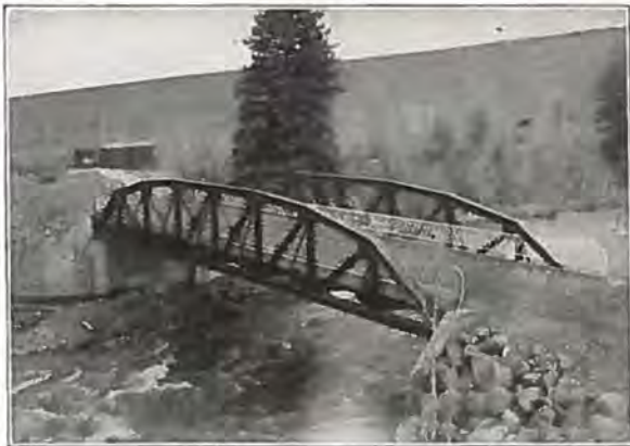
100 ft. Riveted Low Truss Span, Dillon, Colo.
