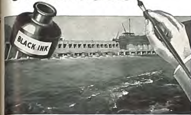
View showing $25,000,000 Rock Island, Wash., Hydro-Electric development in Columbia River nearing completion. One solitary No. 300W Pioneer Washing, Screening, Crushing and Loading Plant, owned and operated by L. Romano Engineering Corporation of Seattle, produced all the coarse aggregate and sand required for this huge job.
