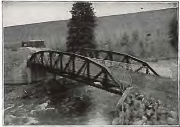
100 ft. Riveted Low Truss Span, Dillon, Colo.
