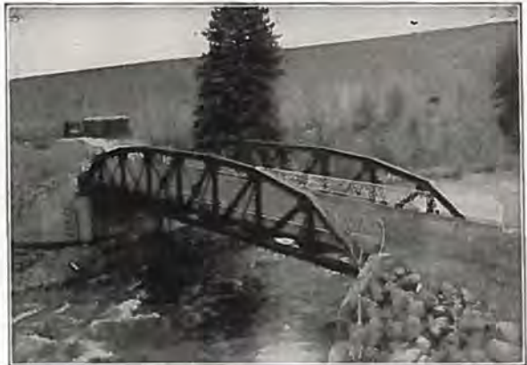
100 ft. Riveted Low Truss Span, Dillon, Colo.
