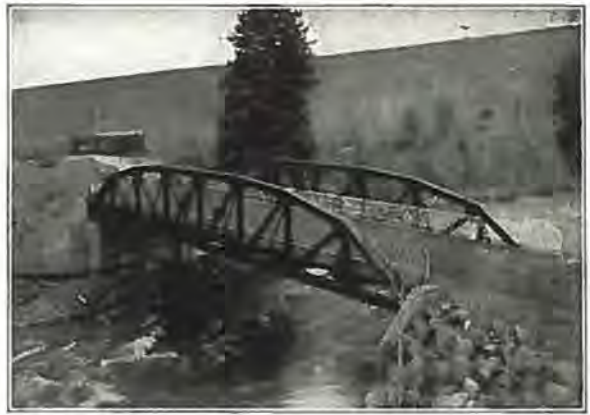
100 ft. Riveted Low Truss Span, Dillon, Colo.
