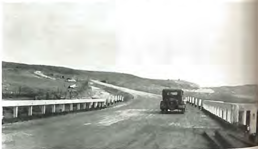
A scene taken along the new gravel-surfaced highway between Fort Collins and Laramie, Wyoming, recently opened to traffic.
