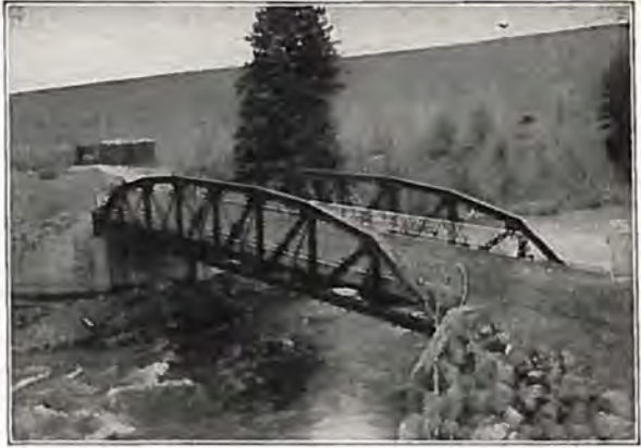
100 ft. Riveted Low Truss Span, Dillon, Colo.
