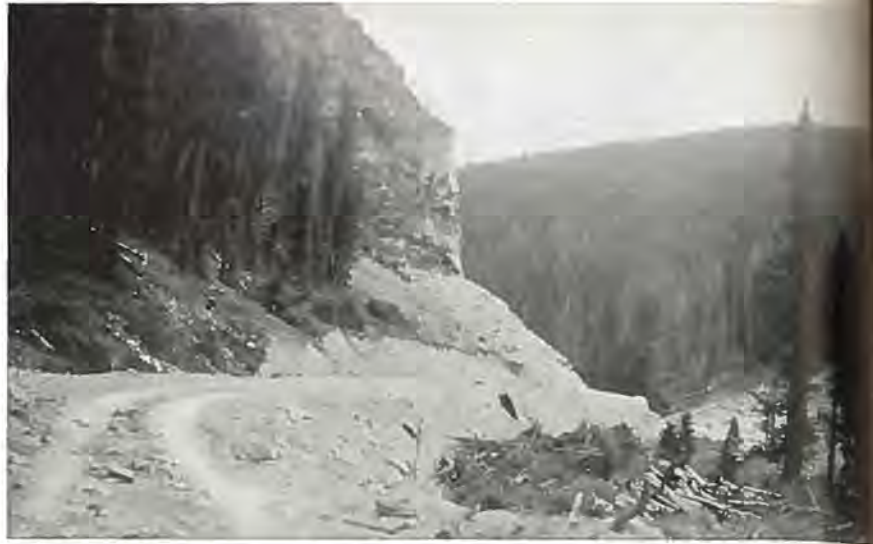
Looking south from the summit of Willow Creek pass, showing rock dyke which was blasted away to make room for the road, and showing condition of road before finishing. Photos by courtesy U. S. Bureau of Public Roads.
