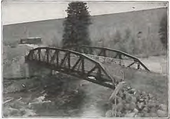
100 ft. Riveted Low Truss Span, Dillon, Colo.
